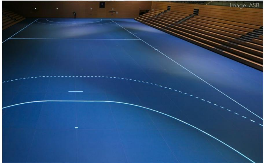
No more confusing jungle of lines in sports halls: printed glass flooring with backlit pitch markings.
